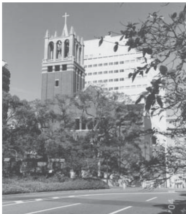
The Kobe Eiko Church, rebuilt nearly 10 years after it was destroyed (photo taken on October 18, 2004, courtesy of Kobe Eiko Church)
