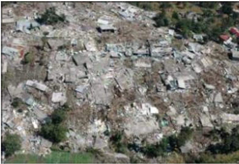
Muzaffarabad after the earthquake
